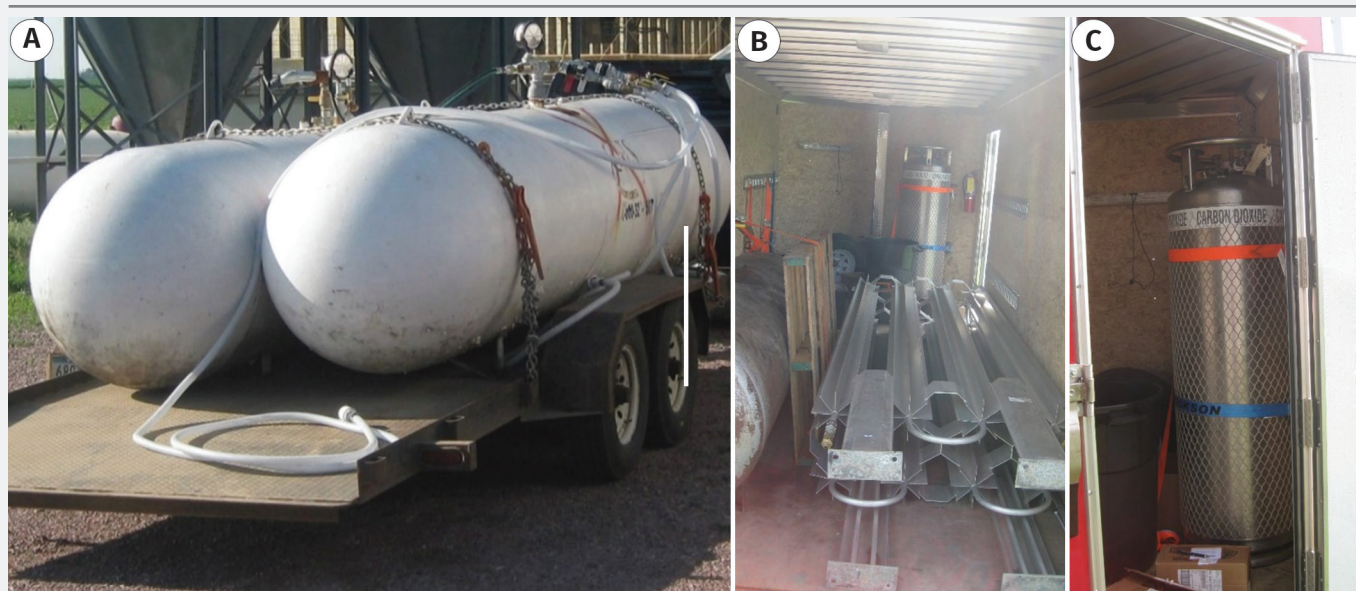
Figure 5: The tanks and non-electric vaporizer used for CO 2 delivery. A) The 1000-gallon low-pressure tanks that flowed CO 2 into the trailer. B) The non-electric vaporizer and C) vertical gas-liquid tank carried on an enclosed trailer and used to fill the low-pressure tanks.
